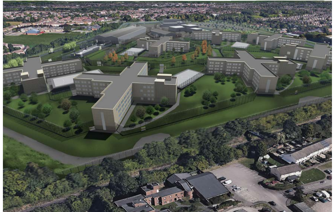
Our new Glen Parva prison in Leicestershire, currently under construction
