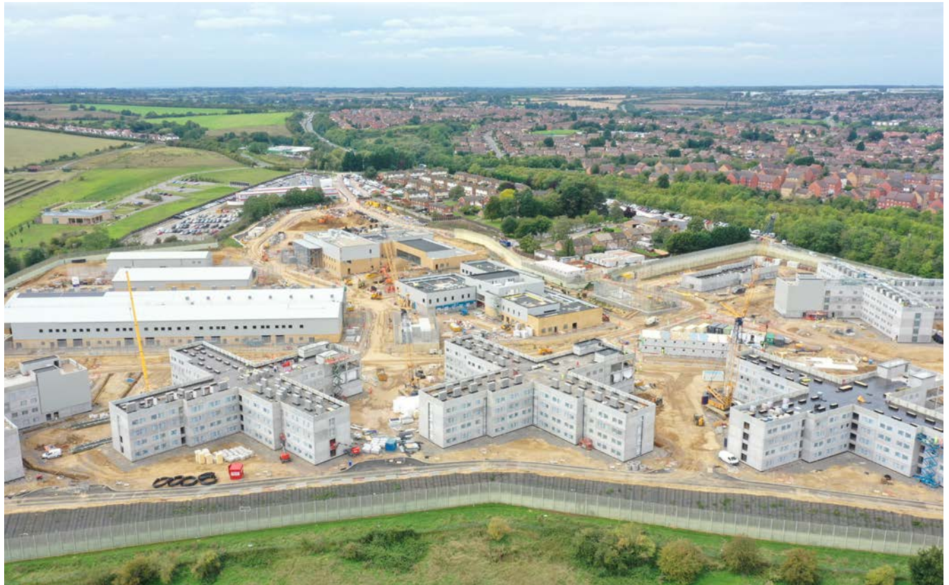
New prison at Wellingborough, HMP Five Wells, under construction
